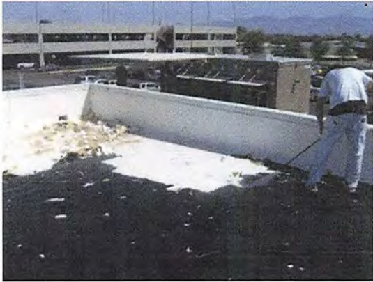
Pressure Washer Removing Elastic Coating
