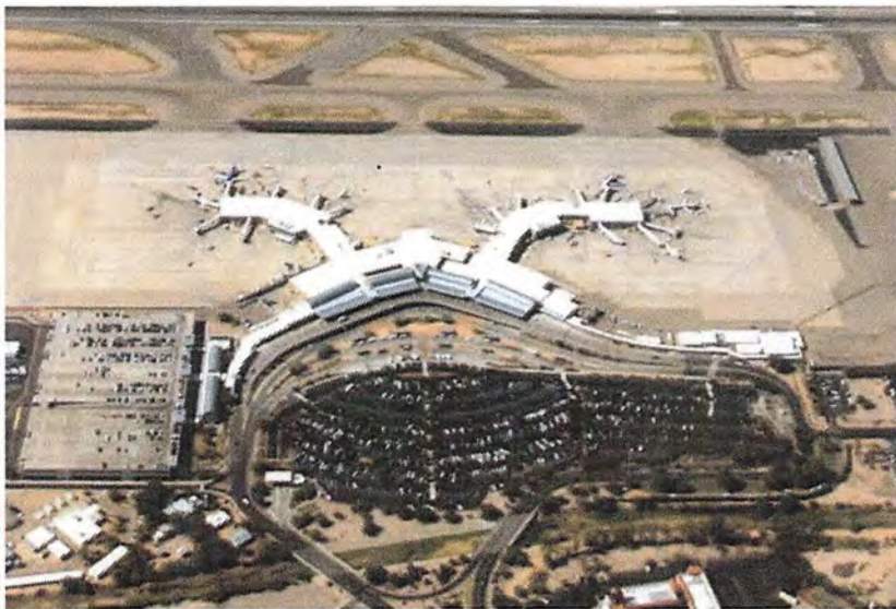
Finished Coating Of Airport Terminal
