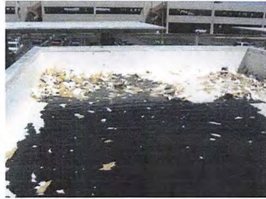
Elastic Coating removed by pressure washing
