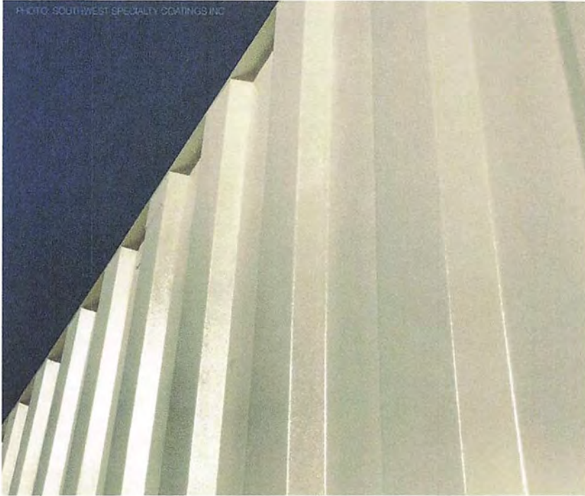
The new coating reflects rather than absorbs heat from the sun.
