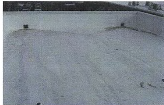
Roof Before Pressure Wash
