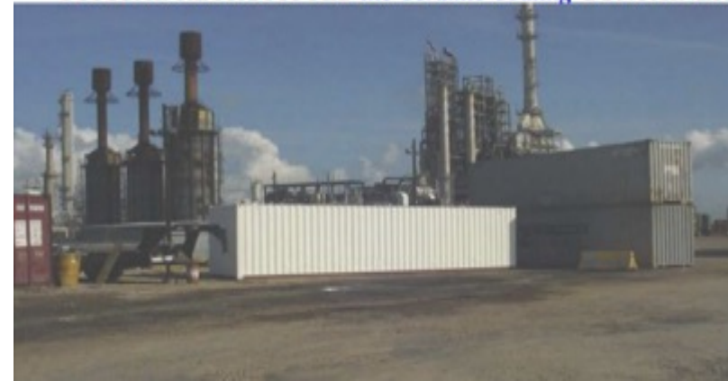
TYPICAL RETROFITTED the Ceramic Coating CONTAINER
