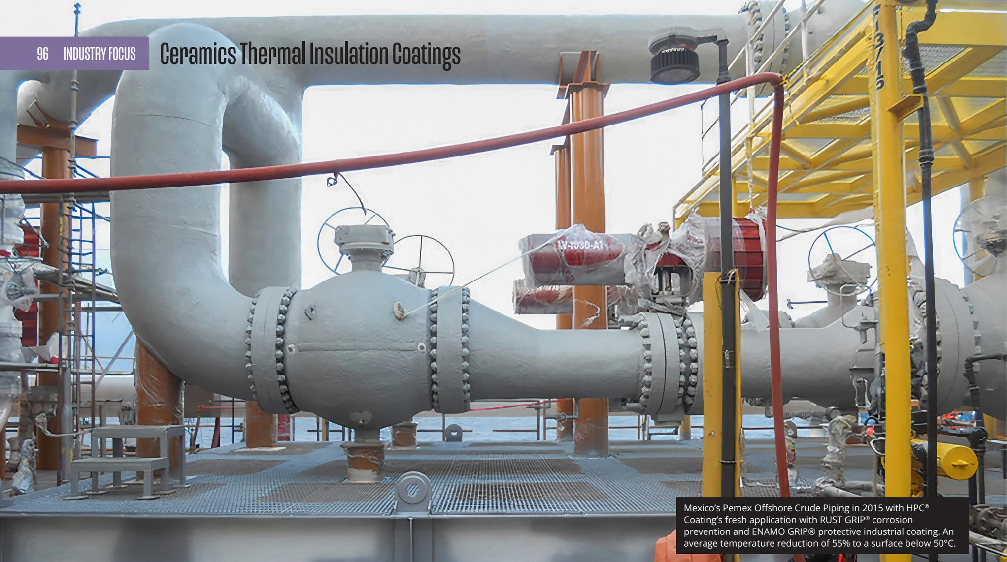
Mexico's Pemex Offshore Crude Piping in 2015 with HPC® Coating's fresh application with RUST GRIP® corrosion prevention and ENAMO GRIP® protective industrial coating. An average temperature reduction of 55% to a surface below 50°C.
