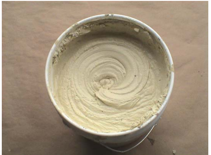
HPC – After Proper Mixing / Ready to Apply
