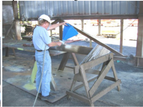
A temperature reduction from 350C on the bare pipe to 170C after the initial primer coat @ 50 mils (1.2mm) DFT was applied.
