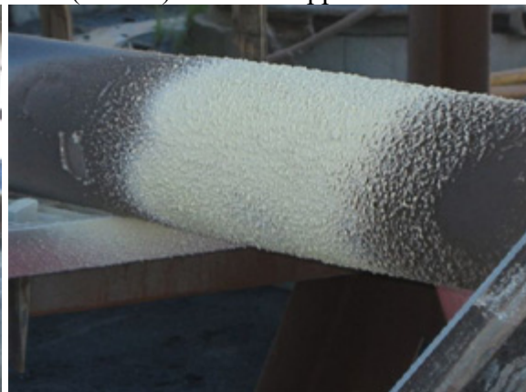
A temperature reduction from 370C on the bare pipe to 90C after the second primer coat @ 50 mils (1.2mm) DFT was applied. ( Video )
