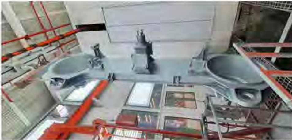
RUST GRIP® maintains an extremely low permeability. This eliminates the penetration of moisture, salts, and acids and the opportunity for corrosion to develop. Bogie bolster being coated with Rust Grip at RCNK
