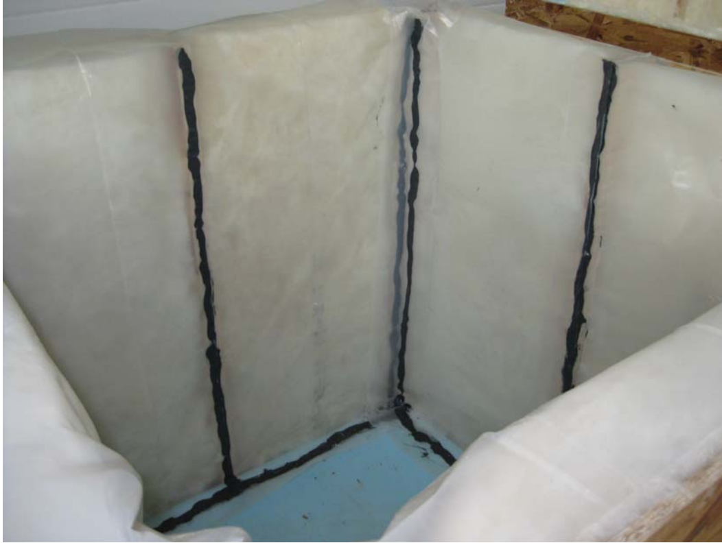
Figure 2. Picture of box construction before the gypsum board was added
