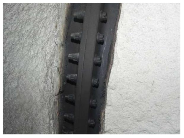
In some cases, Insulative Coatings can be applied over fiberglass or rockwool wrapped around bolts which can then be cut to expose the bolts if needed.
