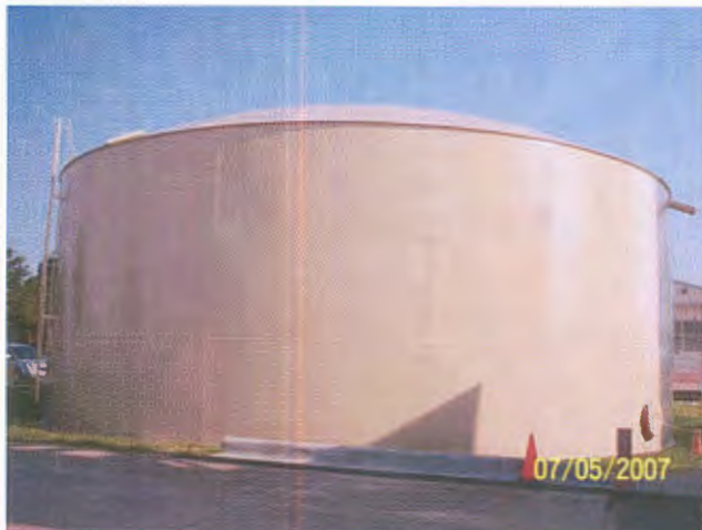
Pictures of the domed-roof deluge tank and the aircraft hangar at Simmons Army Airfield AFTER the Rust Grip/Enamo Grip application.
