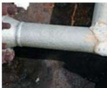
*Corrosion Under Insulation*
